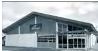
Further production facilities of A. Schweiger GmbH, Sauerlach near Munich
